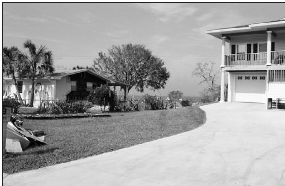
Figure 17. Post-hurricane photo showing elevated building surrounded by gently sloping fill, with adjacent damaged pre-FIRM building (the presence and configuration of the fill were judged by the damage inspection team not to have led to flood or wave damage to the elevated building or the nearby pre-FIRM building).
