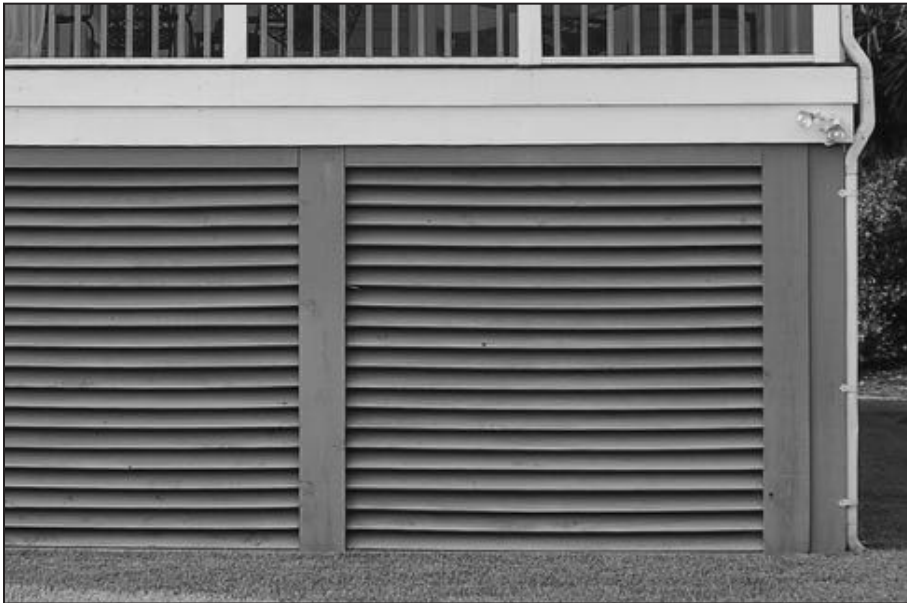
Figure 5. Wood slats installed between pilings at an angle (louvers)
