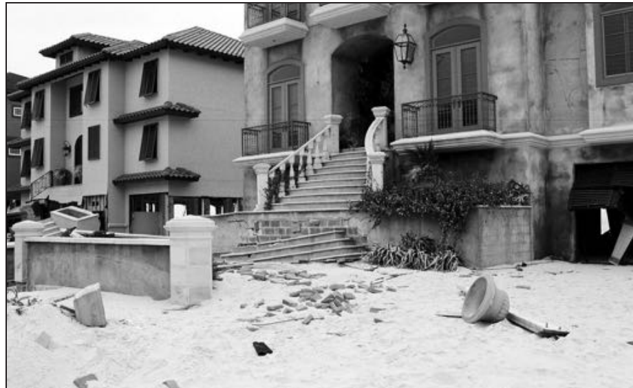
Figure 3. Massive stairs adjacent to an elevated coastal home are an obstruction.
