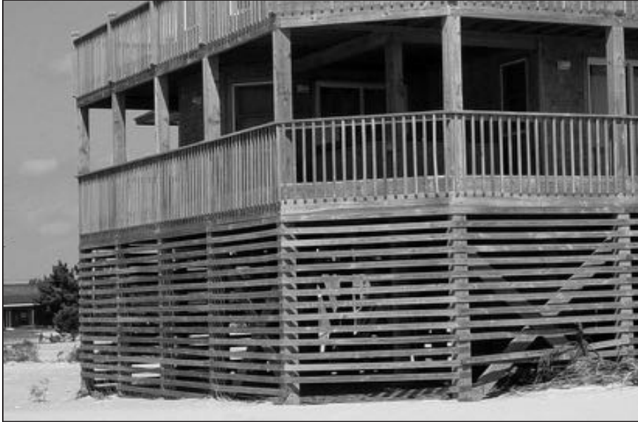
Figure 4. Wood slats installed flat against foundation pilings
