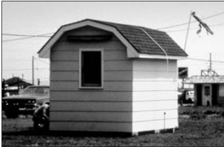
Figure 14. Small accessory structure anchored to resist displacement by wind
